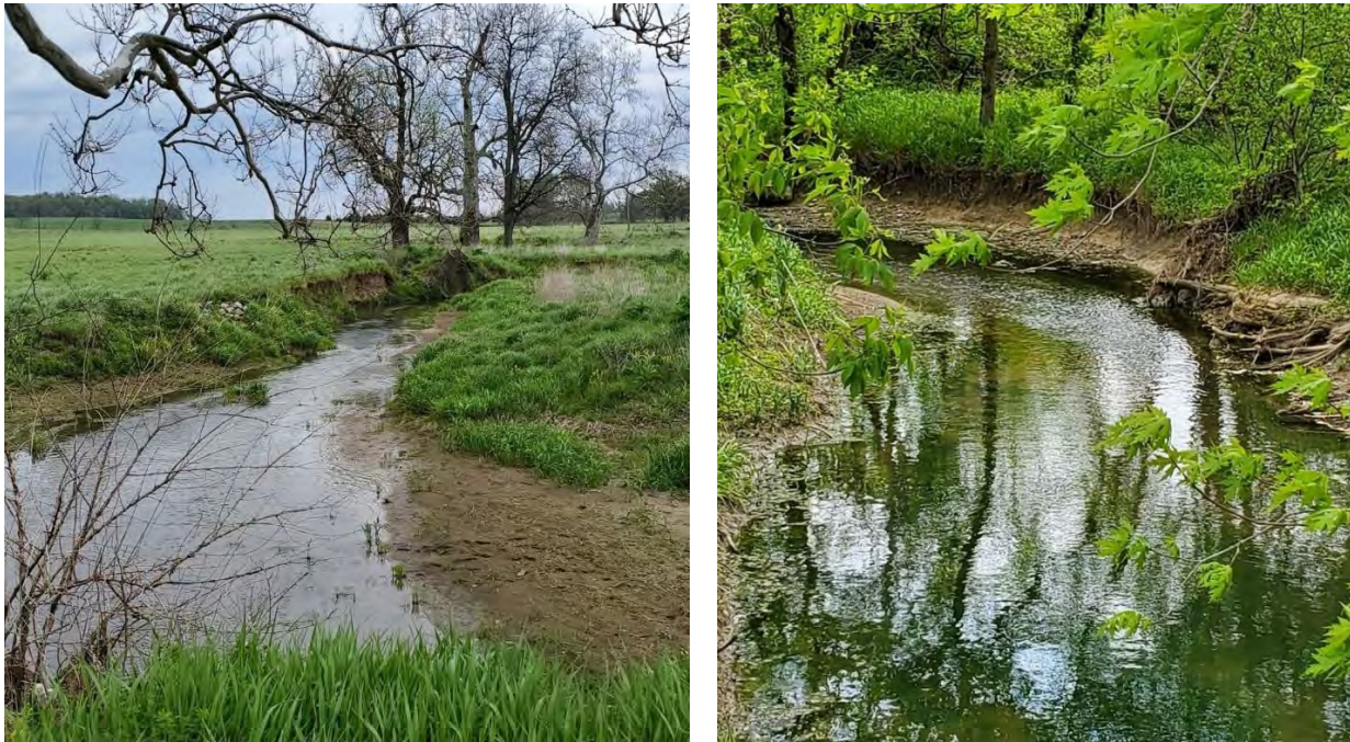
Figure 55. Streambank erosion observed throughout the Walnut Fork-Sugar Creek Watershed.
